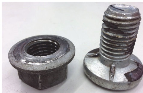
Figure 8. A bolt and nut after dismantling
