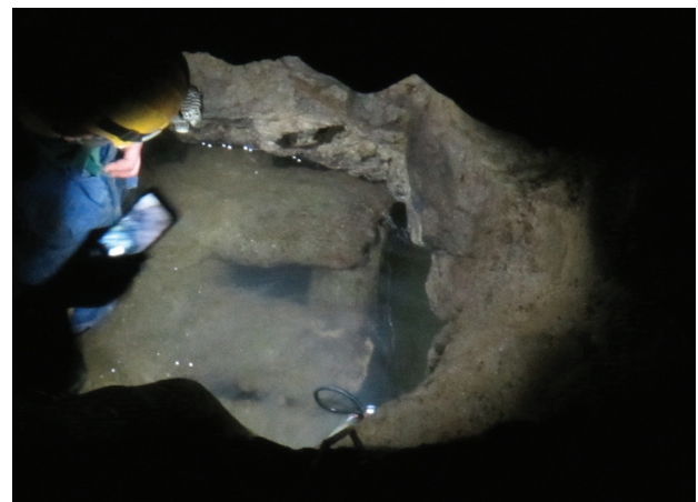
Fig. 7. Bystrzyca Górna, site 26. End section of the shaft examined in 2017 with visible elements of wooden lining connecting it with the central drift (photo by T. Stolarczyk)
