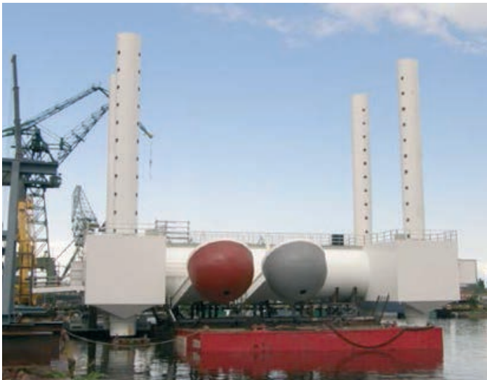
Fig. 4. Wave Star offshore wave plant module during outfitting at Gdańsk Shipyard (2009)
