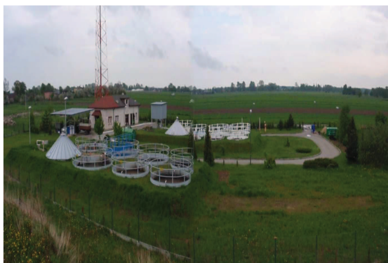
Fig. 1. The view of the developed wastewater treatment plant in Dobron
