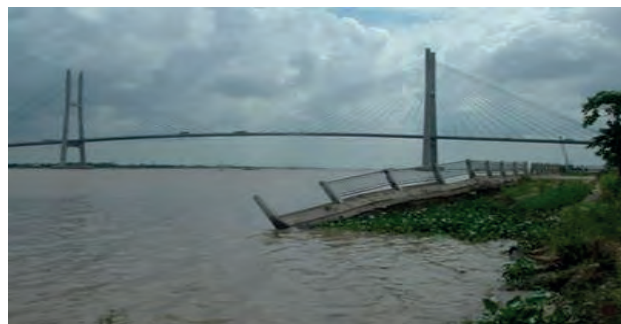
Figure 2. Riverbank erosion of the Tien River, near to the My Thuan Bridge
