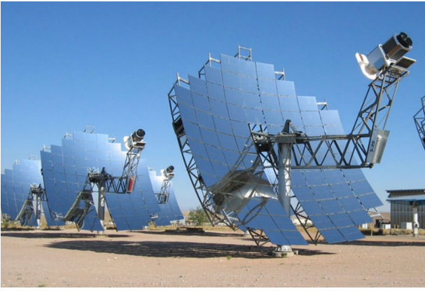
Fig. 3. The solar power plant using Stirling engines [8]
