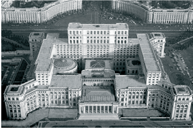
Fig. 7. Spatial symbol of political power constructed by N. Ceausescu: Palace of Parliament (originally People's House), 1984-1997, Bucharest, Romania. This neoclassical building is the world's largest and most expensive civilian building 1 .
