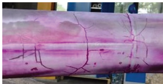
Fig. 1. The appearance of the pipe after penetration tests
