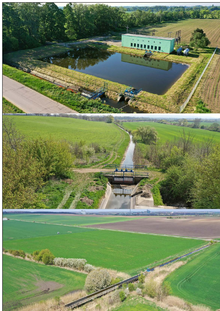
Figure 8. Water reservoir and water filling station (up), regulation device on the irrigation canal Krhovice-Hevlín (middle), historic aqueduct on the Krhovice-Hevlín irrigation canal (down)
