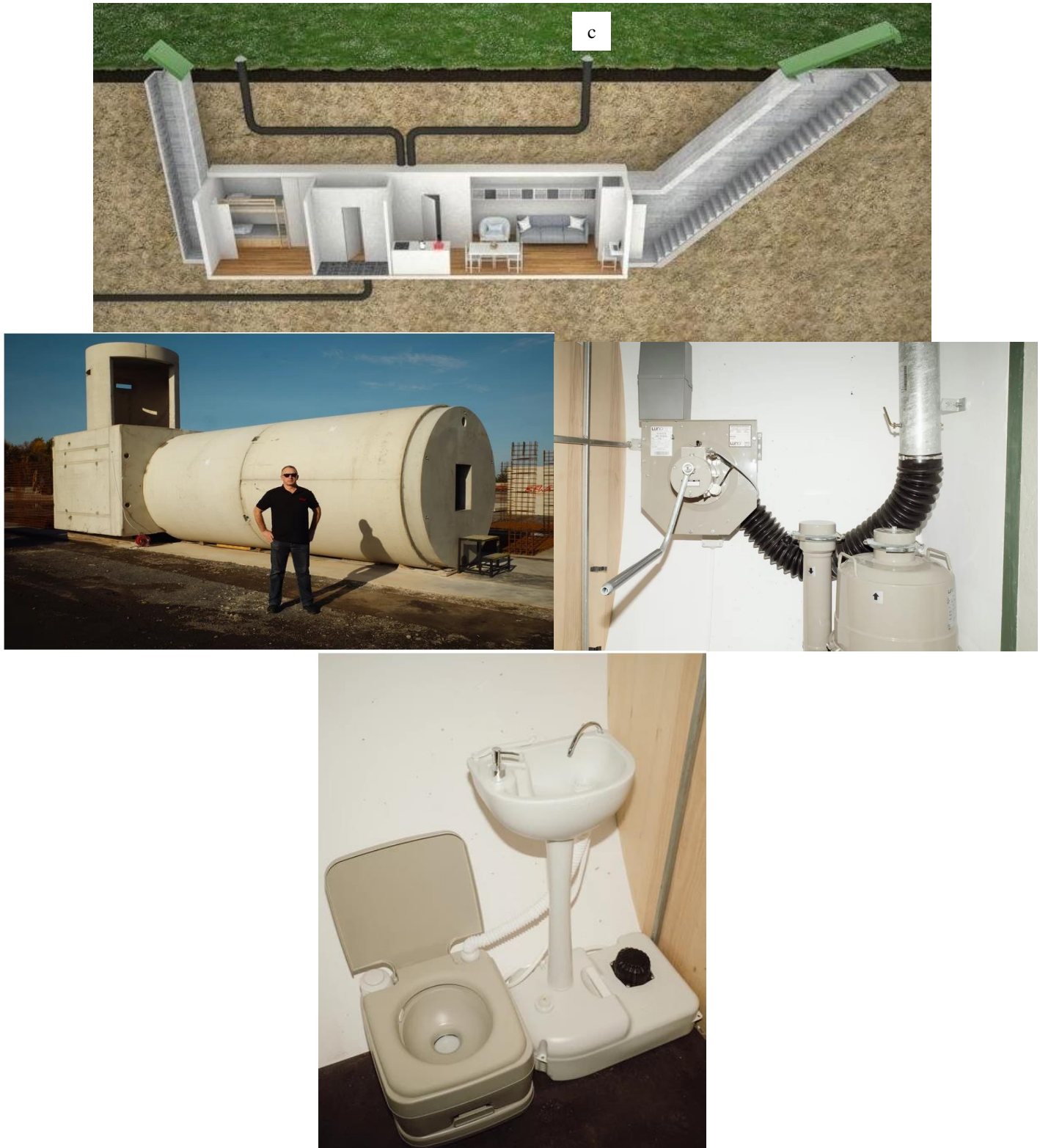
Fig. 11. Family backyard shelter (a) hiding scheme, (b) a demonstration home shelter that buries from 2 m to 6 m underground, (c) an eclectic (12V) and hand-powered filtration system, (d) a portable sanitation unit powered by a hand or electric pump [25].
