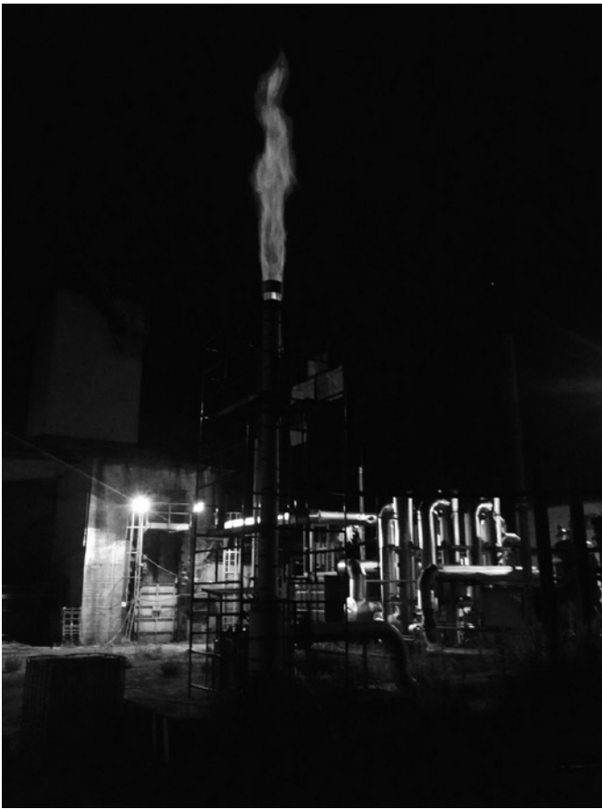
Fig. 8. Flare and part of UCG gas purification system
