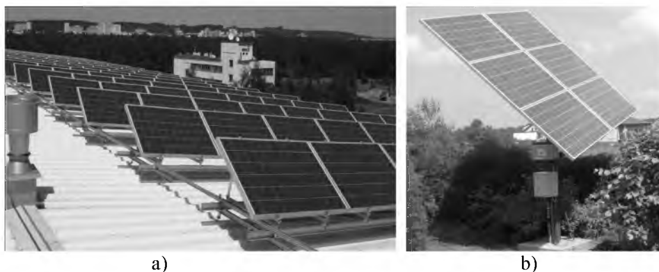
Fig. 1. Examples of photovoltaic installations: stationary on Frosty roof in Bydgoszcz (a), [phot. Grażyna Frydrychowicz-Jastrzębska] and provided with Sun follow-up; the tracker with PV modules (b), the Communication Plant of Alarm System PHU, Leżajsk [with approval of Mr. Stanisław Krupa]
