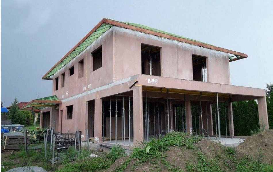
Fig.5. Two-storey house in Gliwice – installation of the roof; authors' own photographs
