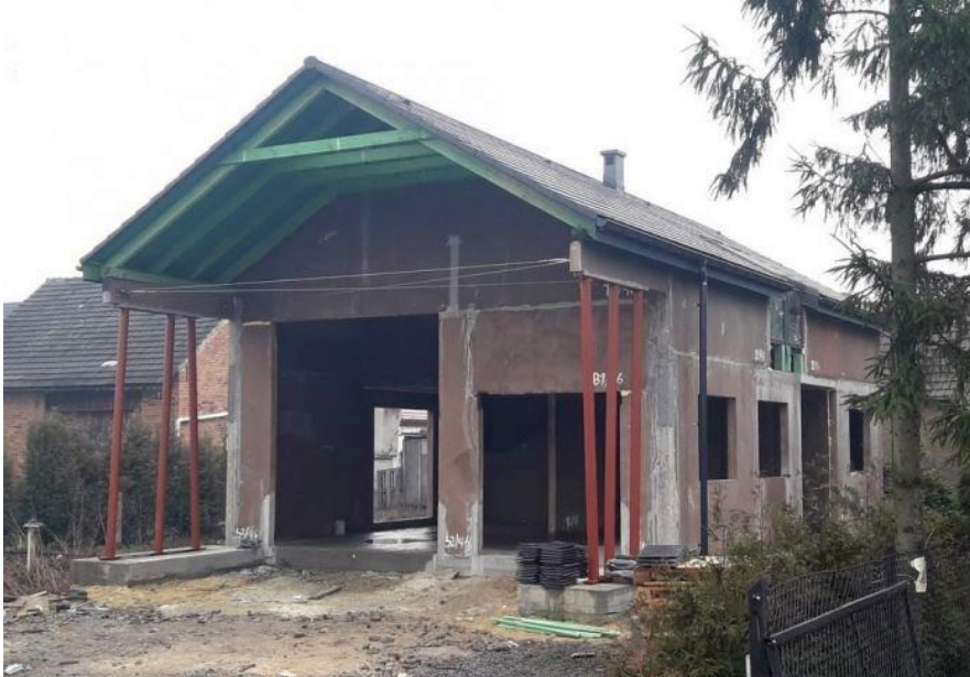
Fig. 7. Two storey house in Wry – construction site; authors' own photographs
