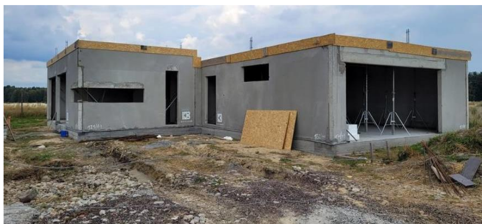
Fig. 3. Single-storey house, Rachowice - photo during wall installation, authors' own photographs
