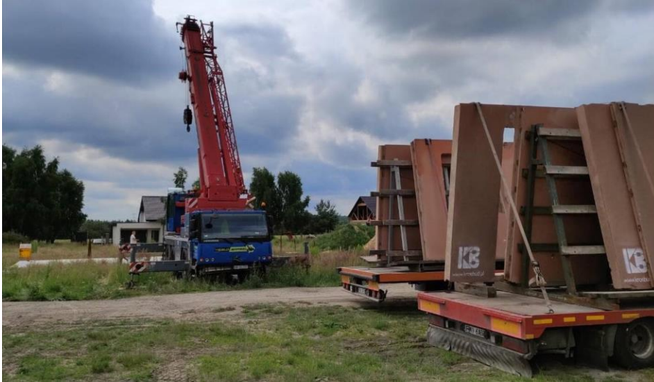
Fig. 2. Expanded clay concrete panels, authors' own photographs
