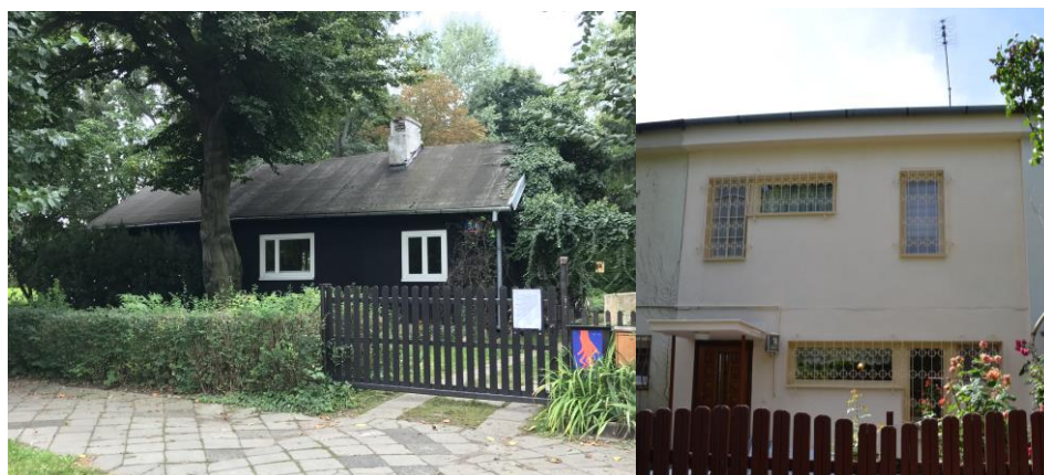
Fig. 1. Warsaw prefabricated Finnish houses (1945) and row houses in the Prototypy estate (1960s, today additionally insulated), authors' own photographs
