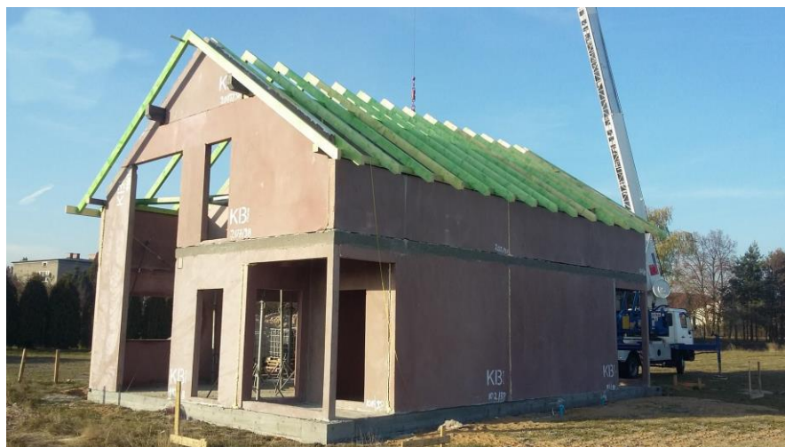
Fig. 6. Two-storey house in Wry – installation of the roof; authors' own photographs
