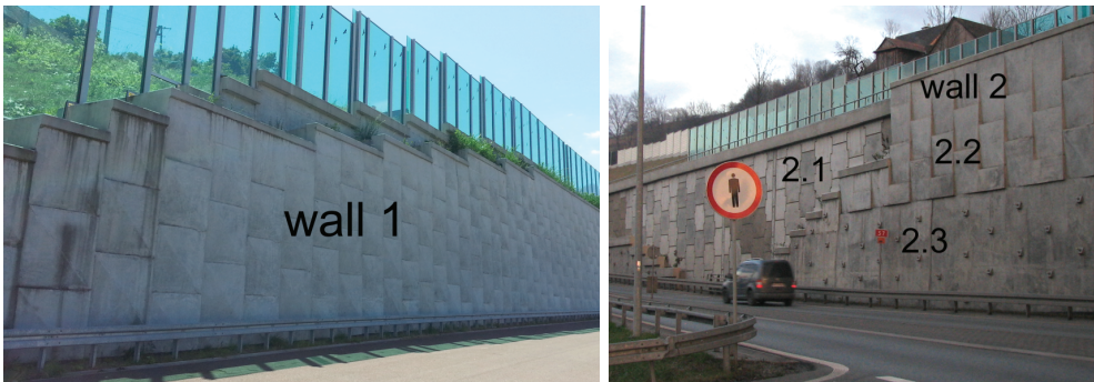
Fig. 2. Fragments of the retaining walls subject to the surveys
