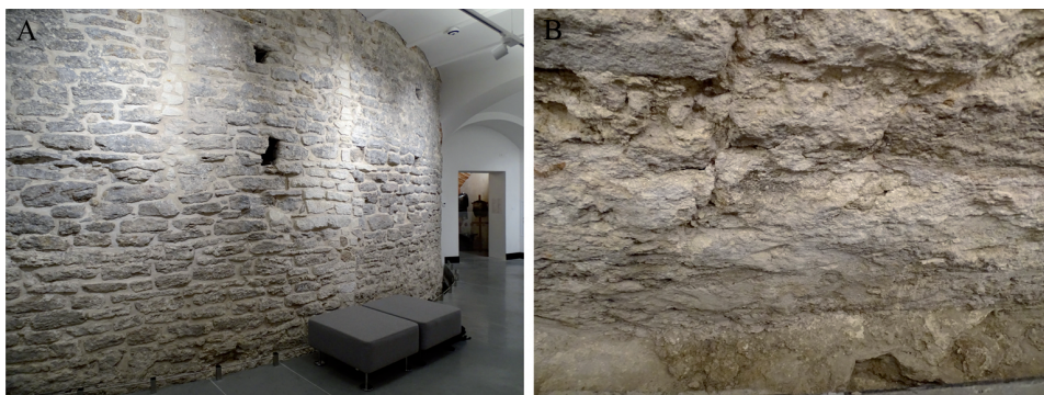
Fig. 2. A) Stone part of the cylindrical tower in the first floor of the south wing of the Lublin Museum building, B) Stone arrangement in the face of the cylindrical tower visible from the first floor of the south wing of the Lublin Museum building
