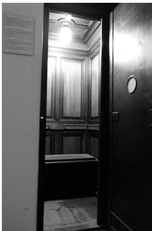
Fig. 1. Electric passenger elevator in former Landeshaus der Provinz Silesia in Breslau (now the headquarters of the Supreme Technical Organization) from 1897, manufactured by Carl Flohr Berlin company (photo by K. Pietrzak)
