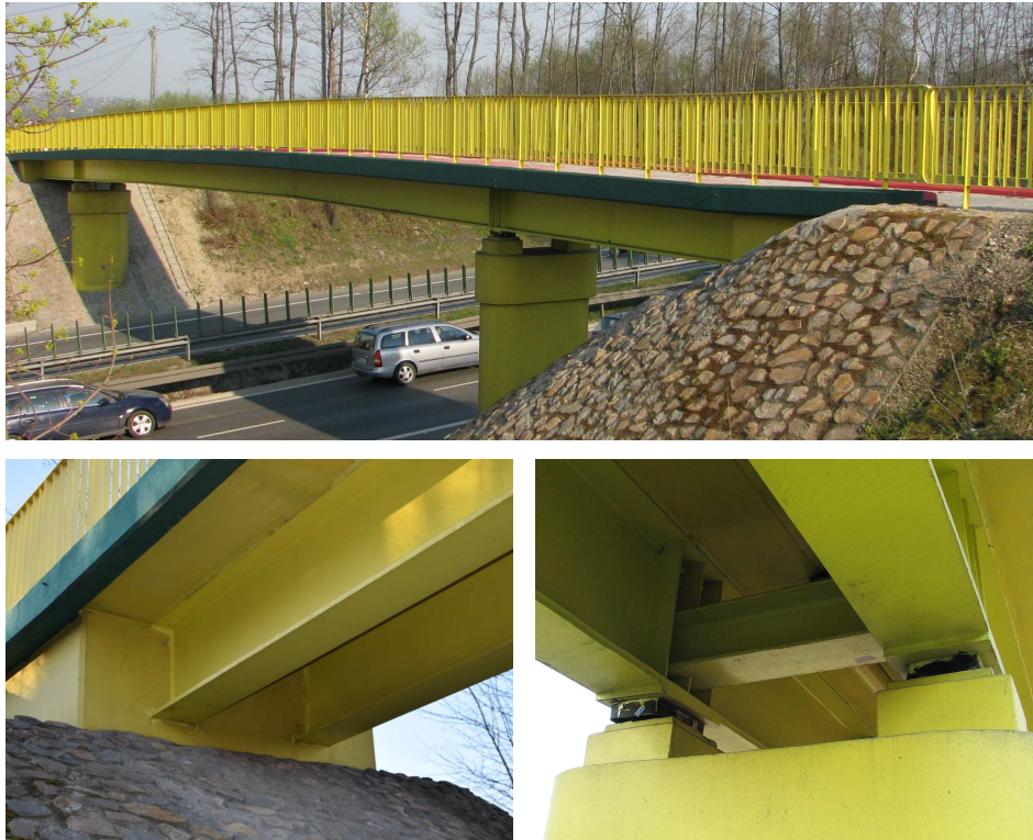
Fig. 3. General view of the footbridge and selected details
