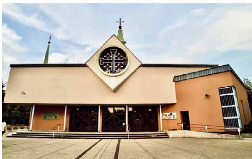
Fig. 1. Św. Jerzy Church in Poznań – view of the building; source: author
