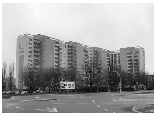
Fig. 8. Kalina II estate, residential building, XII-floors, 10-entrance, project 1977, current state.
