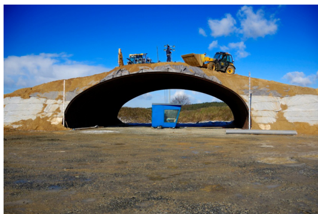
Figure 1: Loads occurring during the construction of soil-steel structure.
