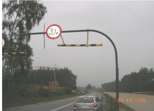
Fig. 7. View of beam marking height of clearance (3.70 m) before entry into the road section where scaffolds were being erected and reinforcement installed prior to casting spans (vertical clearance for all viaduct being built was 4.20 m and was larger than clearance height on warning gate where there was exit leading to another road).
