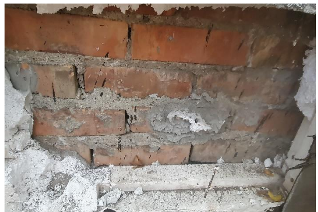
Photo. 9: View of the outer wall (from the escarpment side) of the former office rooms (A): a) O1, b) O2, c) O3, d) O4, e) O5, f) O6, g) O7, h) O8, i) O9, j) O10, k) O11
