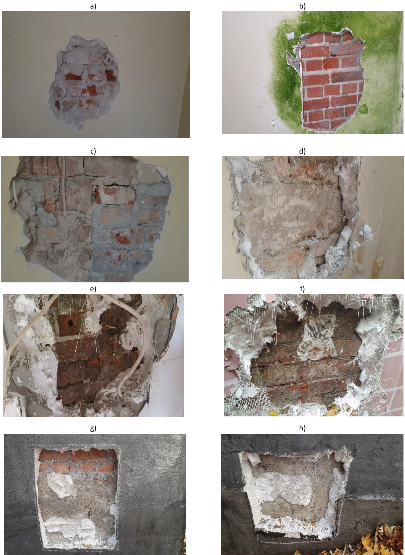
Photo. 9: View of the outer wall (from the escarpment side) of the former office rooms (A): a) O1, b) O2, c) O3, d) O4, e) O5, f) O6, g) O7, h) O8, i) O9, j) O10, k) O11
