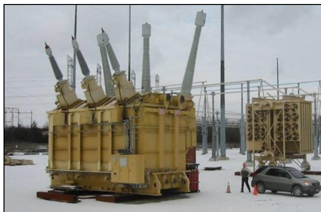
Rys. 9. Transformator 750MVA po suszeniu LFH Fig. 9. UHV 750 MVA Transformer after LFH drying
