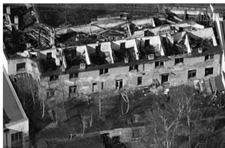
Fig. 3. The top view of the complex of the dry cleaning service "Rainbow" before the demolition, after the fire, around 2012, Source: googlemaps, 06.03.2014]
