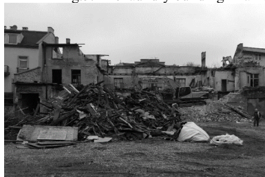
Fig. 6. The segregation of materials from the demolition of the building, Source: own photo, 03 - 04.2014
