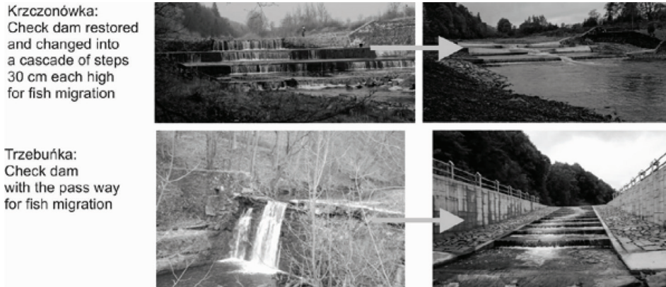
Figure 2. Check dams lowering: Krzczonówka and Trzebuńka Streams (Photos: M.Łapuszek., Ab Ovo Association).
