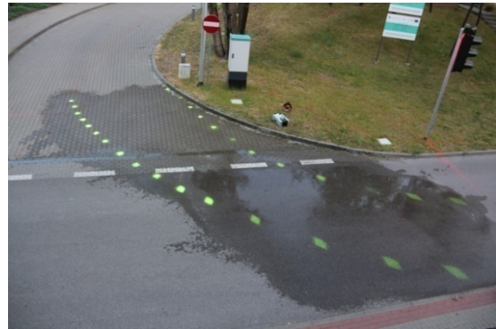
Fig. 6. The visibility of the SPIKer system dots on the wet road
