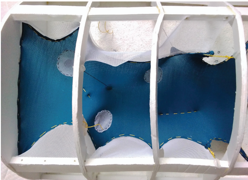
Fig. 4. Additional security net to protect the user from falling off the platform or falling into the "funnel" of the membrane. "Funnels" are a characteristic form of membrane surfaces and take the form of sudden lowers of the diaphragm to tension it and give it a rigid, two-curved surface. Author: A. Olszewska
