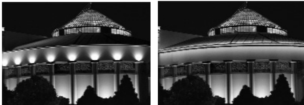
Fig. 1. Different appearance of a wall as a result of different luminance distributions [photo W. Żagan]
