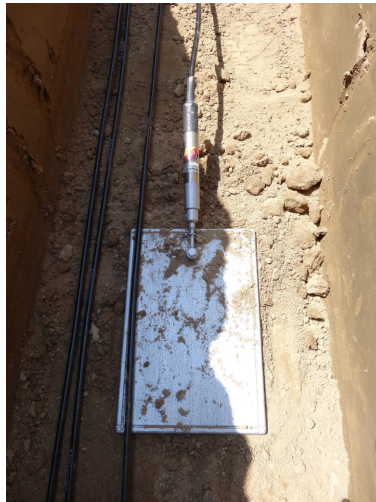
Figure 5. Installation of earth stress sensor [4].
