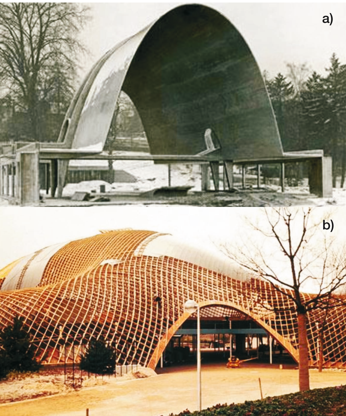
Fig. 1a–b. Shell structures, a) Robert Maillart, Cement Hall, Zurich National Exhibition, 1939, b) Frei Otto, Carlfried Mutschler, Joachim Langner, Multihalle, Mannheim, 1975; source: Debney P. (2015).
