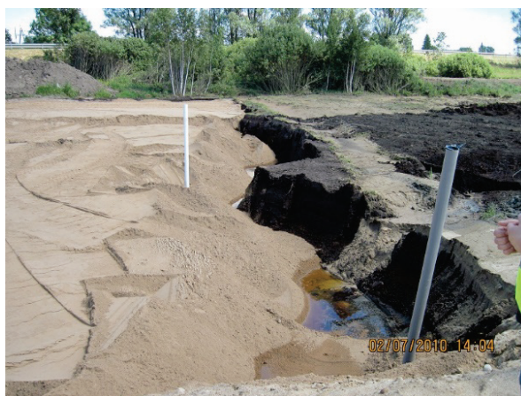
Fig. 4. Replacement of low-bearing capacity soil [8]
