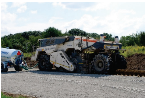
Fig. 2. Chemical stabilization of the soil subbase [8]
