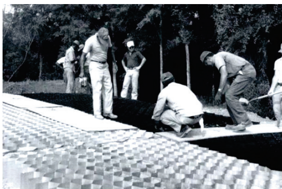
Fig. 9. Testing the efficiency of geocells made of plastic and aluminium (WES, Vickburg, Missouri, 1979) [15]
