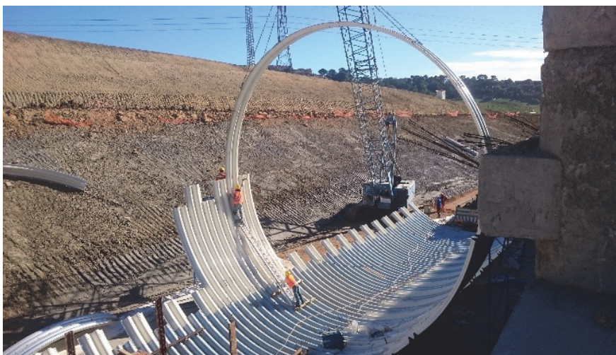
Fig. 9. Assembly of the bottom part of tunnel
