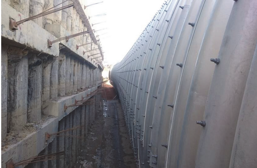
Fig. 12. View from concrete MSE wall side of the tunnel
