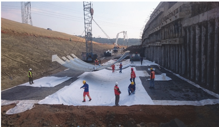
Fig. 8. Bedding preparation before steel structure assembly
