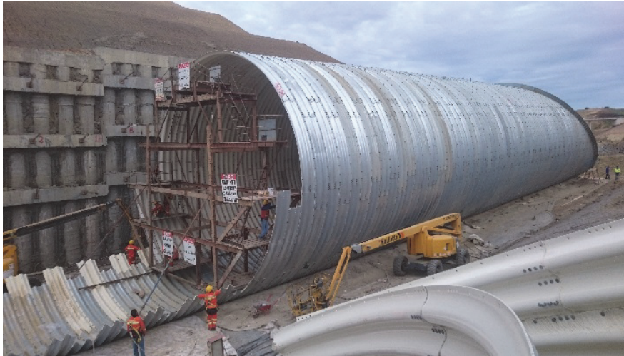
Fig. 10. The assembly with a ring by ring method
