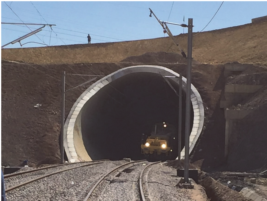
Fig. 13. View from outlet of the completed tunnel
