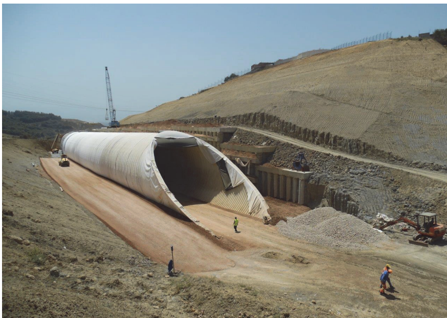
Fig. 11. Instalation of EPDM membrane and nonwoven layers
