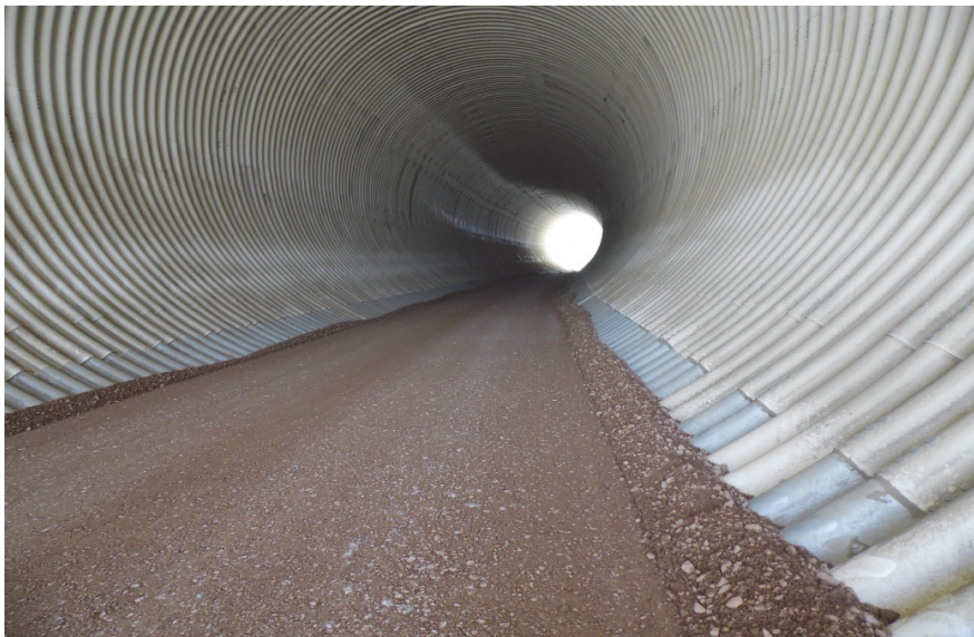
Fig. 12. Inside view , ballast under the rails
