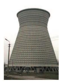
Fig. 5. Prefabricated concrete cooling tower of Darnyts'ka CHP after reconstruction
