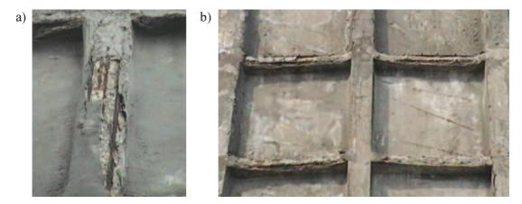
Fig. 2. Some defects in the shell of the cooling tower of the Darnyts'ka CHP: a) corrosion of armature of panel on the vertical ribs, b) corrosion of armature and destruction of the horizontal ribs
