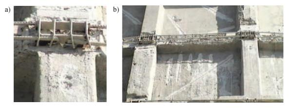
Fig. 4. The process of strengthening performance of horizontal ribs of panels: a) fixation of ring armature on reinforced embedded parts of panels, b) between the embedded parts prestressed reinforcing rods are connected by clamps and fixed to the armature of horizontal ribs
