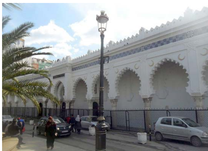
Fig. 1. Djama'a al-Kebir. Algeria
