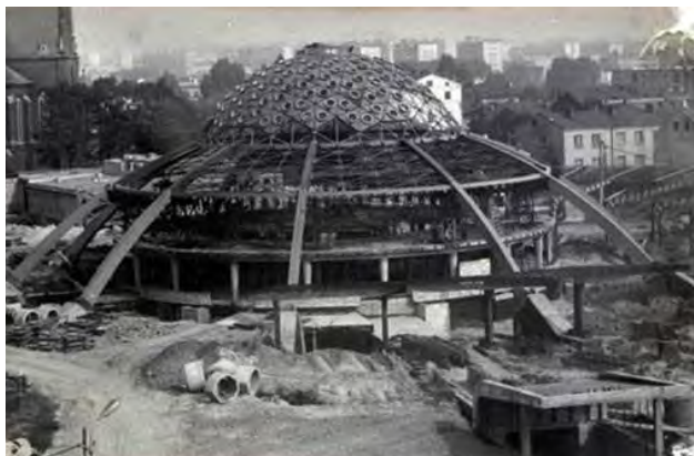
Photo 1. The construction of the new coach station – 1975-1980 (source:Kielce.Wyborcza.pl)
