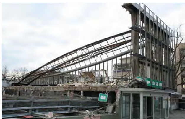
Photo 11. The supermarket during demolition (source: czarnota.org)
