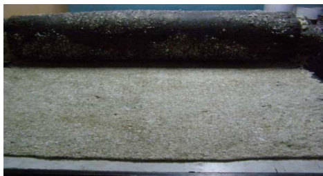
Fig. 8. Non-woven reinforced fabric with grass seed for strengthening slopes and embankments
