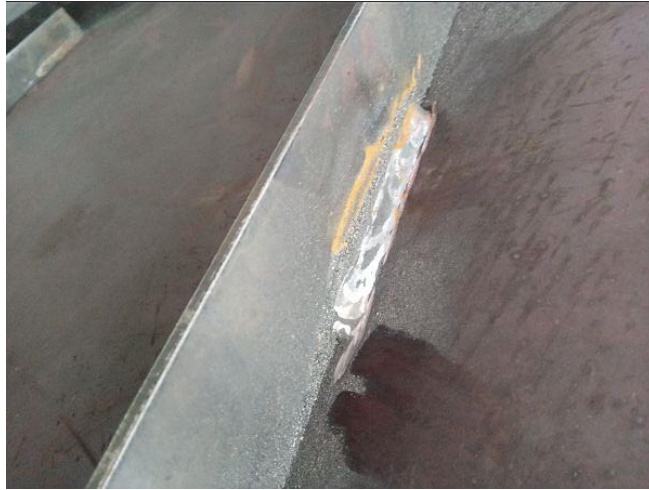
Figure 2. View on the MAG welding (own study).
