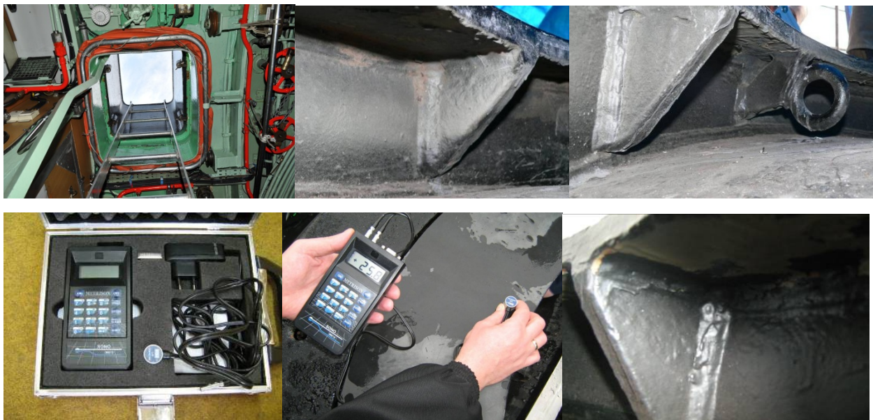
Pic. 3. Pictures of seat area construction during standstill in harbor [2]
