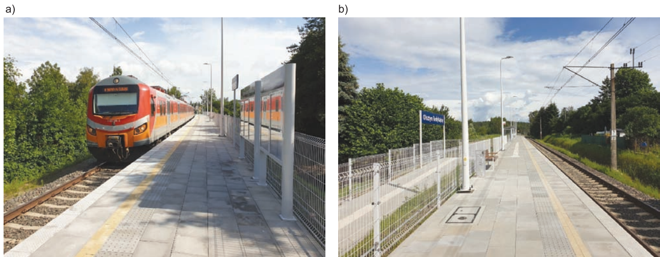
Fig. 6. Lay-by at the Olsztyn Likusy passenger stop [photo: A. Dąbrowski]
