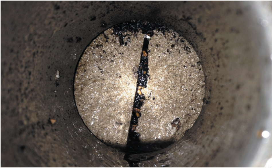
Fig. 13. Fracture opening (1 mm) partially plugged
