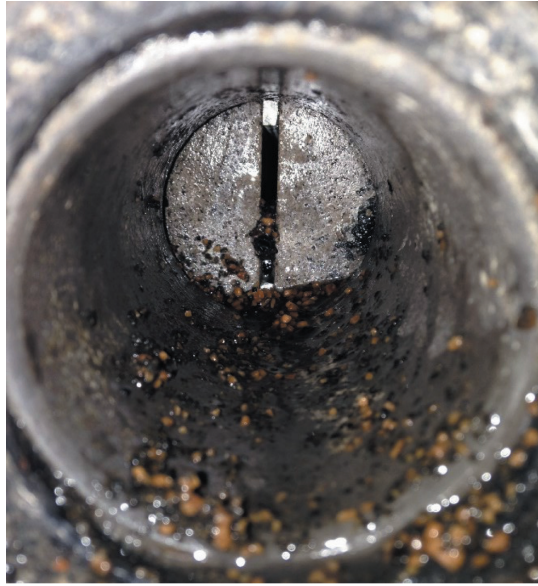
Fig. 15. Fracture opening (3 mm) partially plugged
