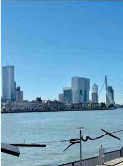
Fig. 10. View at Kop van Zuid district; source: author
