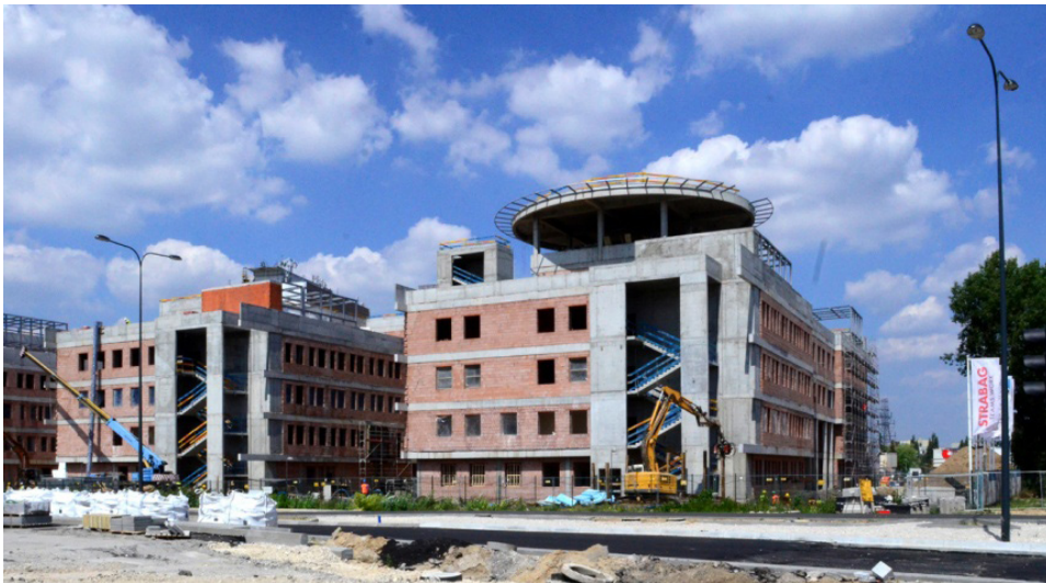
Fig. 1. Helipad on South Hospital in Warsaw under construction. [W. Krzymień, 2018].
