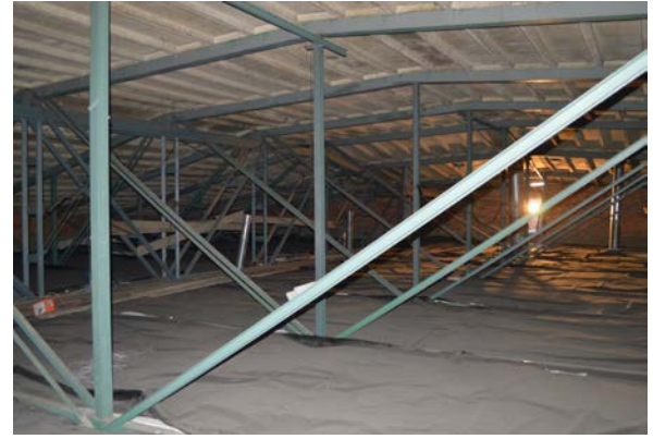
Fig. 10. Inside the ceiling of church VM.
