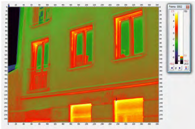
Fig. 2. Thermograph of the multi-flat building
