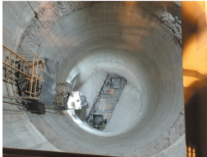
Fig. 5. Construction works in Ore Bunker
