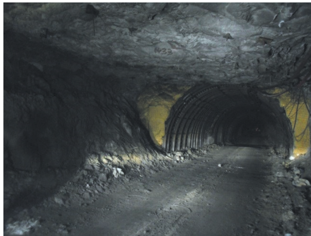
Fig. 4. Drift with Mine roadway supports and EKOFLEX – Mine Foam
