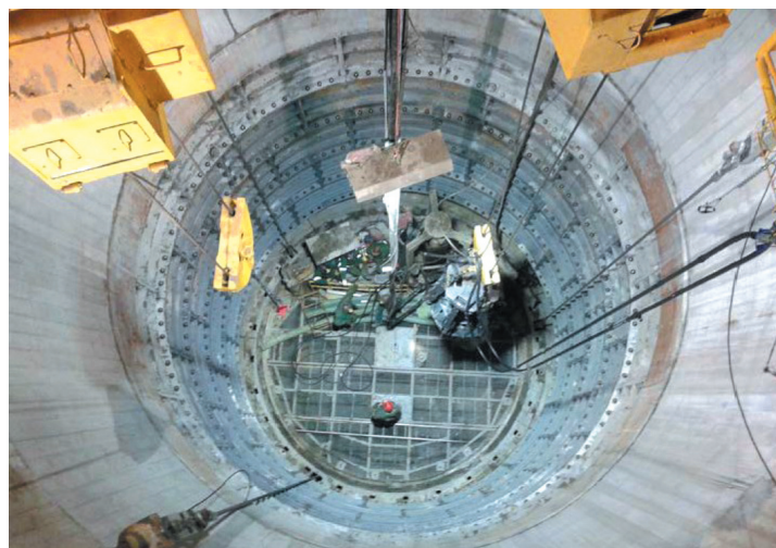
Fig. 2. Sinking the Shaft GG-1 for O/ZG "Polkowice-Sieroszowice" Mine
