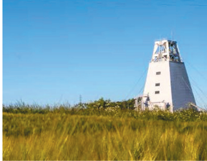
Fig. 1. GG-1 Shaft Tower
