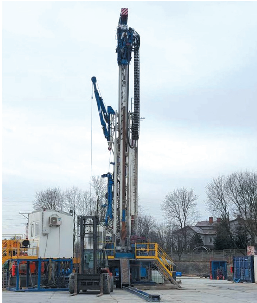
Fig. 6. Geothermal borehole – Tomaszów Mazowiecki
