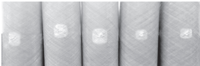
Fig. 7. Damage areas after impact 30 J, visible in daylight [Author, 2015]
