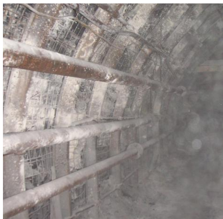
Photo 5. SPL6.8-7.2/3.5/V29 (of S550W steel) support arches built up in gate road 3-Z1,Z2, seam 510/2, Jas-Mos coal mine (Kuziak et al. 2012)
