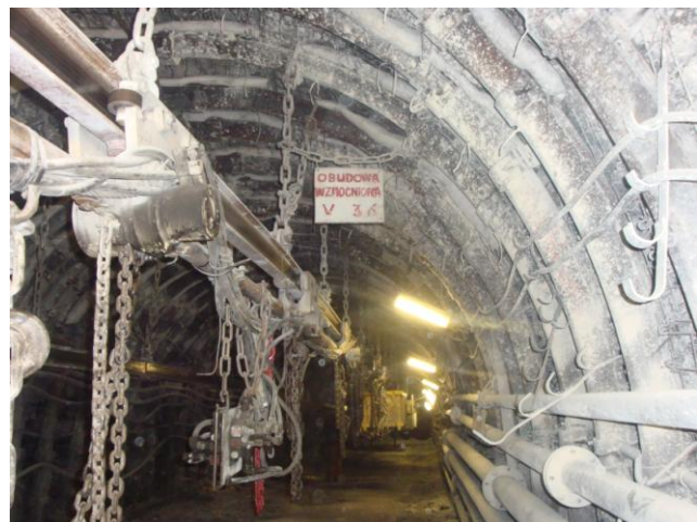
Photo 4. ŁPSC (of S550W steel) support arches built up in gate road 6/VI/385, seam 385, LW Bogdanka SA (Kuziak et al. 2012)
