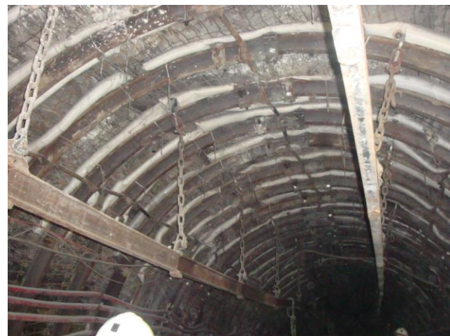
Photo 4. ŁPSC (of S550W steel) support arches built up in gate road 6/VI/385, seam 385, LW Bogdanka SA (Kuziak et al. 2012)
