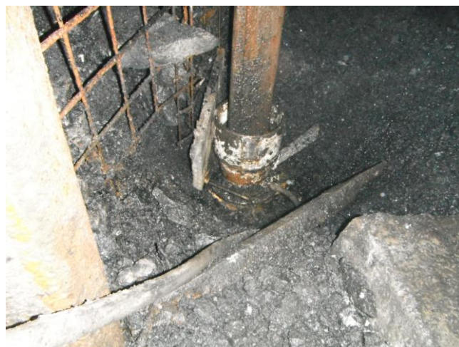
Photo 3. ŁPw support arches built up in test raise 3, seam 504, Bobrek Centrum coal mine (Kuziak et al. 2012)
