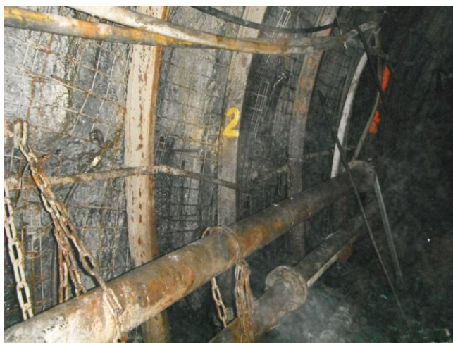
Photo 3. ŁPw support arches built up in test raise 3, seam 504, Bobrek Centrum coal mine (Kuziak et al. 2012)
