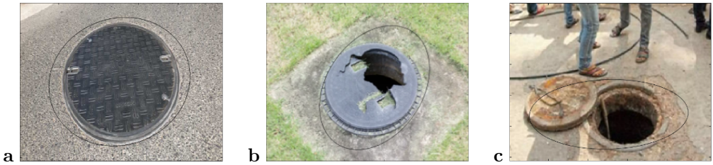
Fig. 5. Samples of the ellipse drawn by the algorithm around each class: (a) closed, (b) broken, and (c) open manhole.
