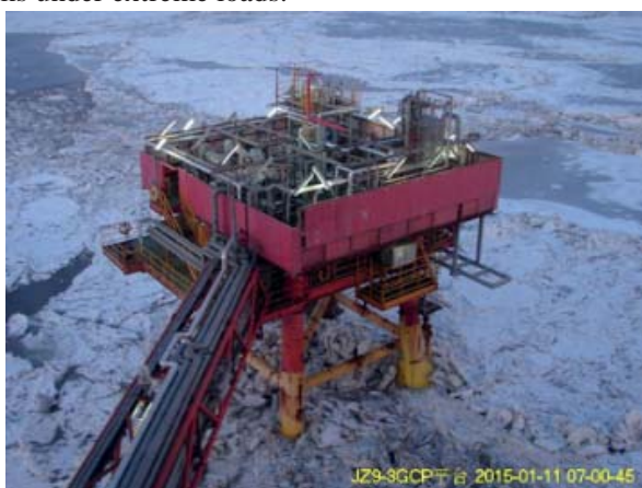
Fig. 2. Typical jacket platform in Bohai Bay
