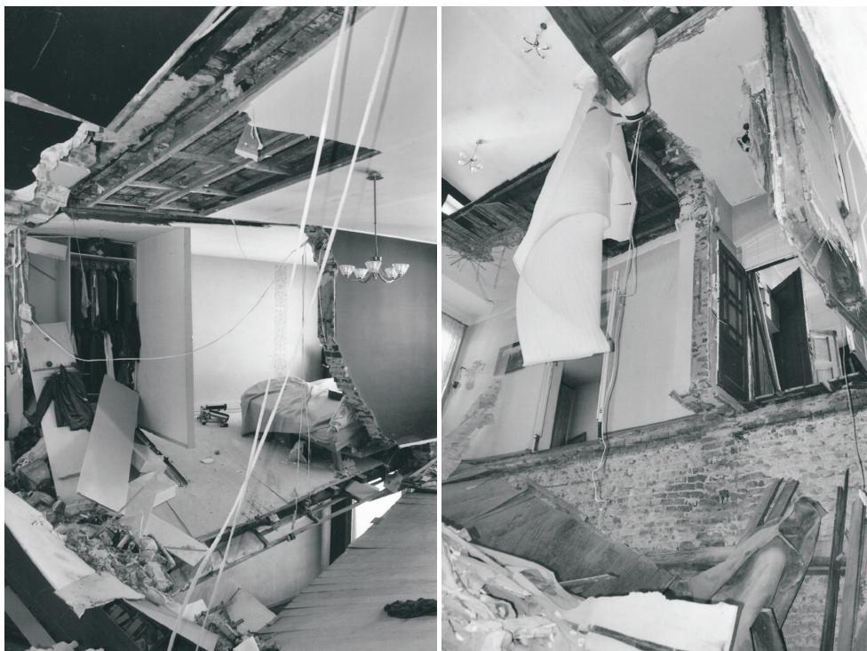
Rys. 2. Fragment parteru i I piętra po katastrofie, widoczny na piętrze fragment ściany w osi „B” Fig. 2. Part of the ground floor and the 1st floor after the catastrophe; a part of the wall in axis „B” is shown on the 1st floor
